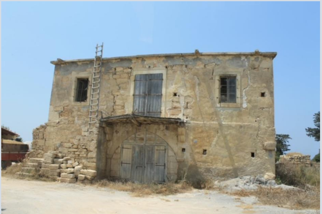
Figure 5 A house still standing up after half a century of hardship.
